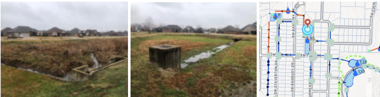
Figure 1. Example of existing stormwater infrastructure at Eden's Brooke and Oxford Ridge. Eden's Brooke and Oxford Ridge stormwater system (City of Bentonville Master Map).
